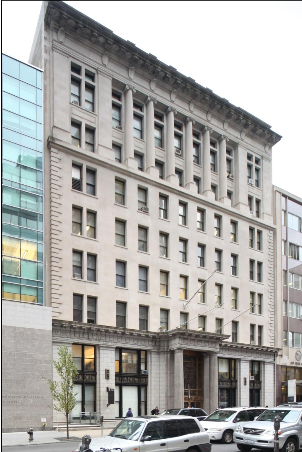
Brooklyn Union Gas Company Building 176 Remsen Street (aka 172-178 Remsen Street) Borough of Brooklyn Tax Map Block 255, Lot 36 in part Built: 1914 Photo: Christopher D. Brazee (2009)
